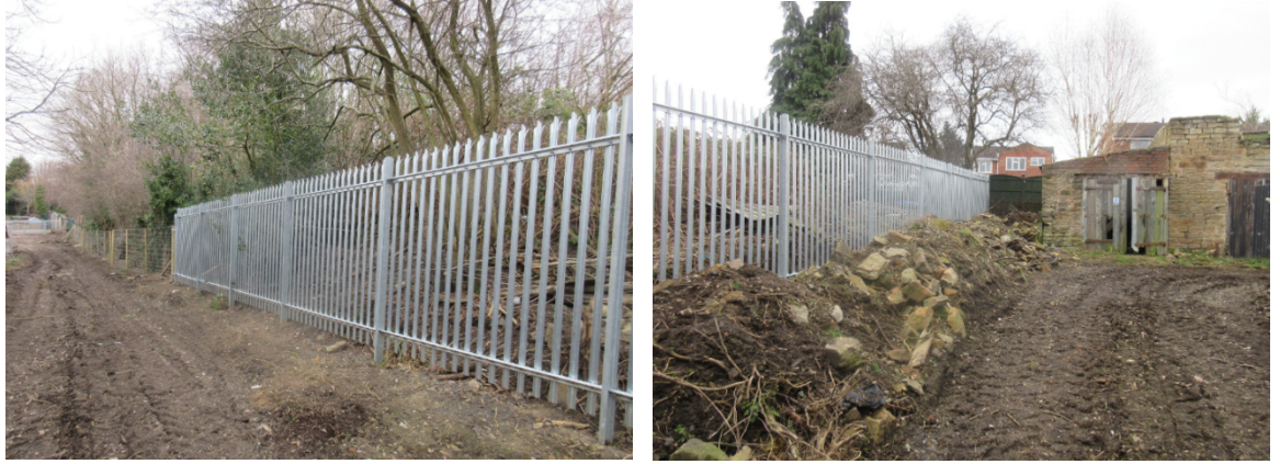
Photographs of fencing in the south eastern corner of the site
