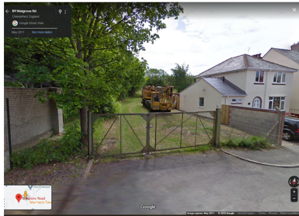
Photographs of fencing and gates on the frontage with Walgrove Road in May 2011
